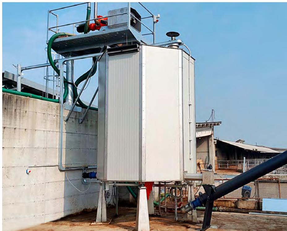
Figure 1 HBC biocell installed with solid/liquid separator and unloading screw conveyor
